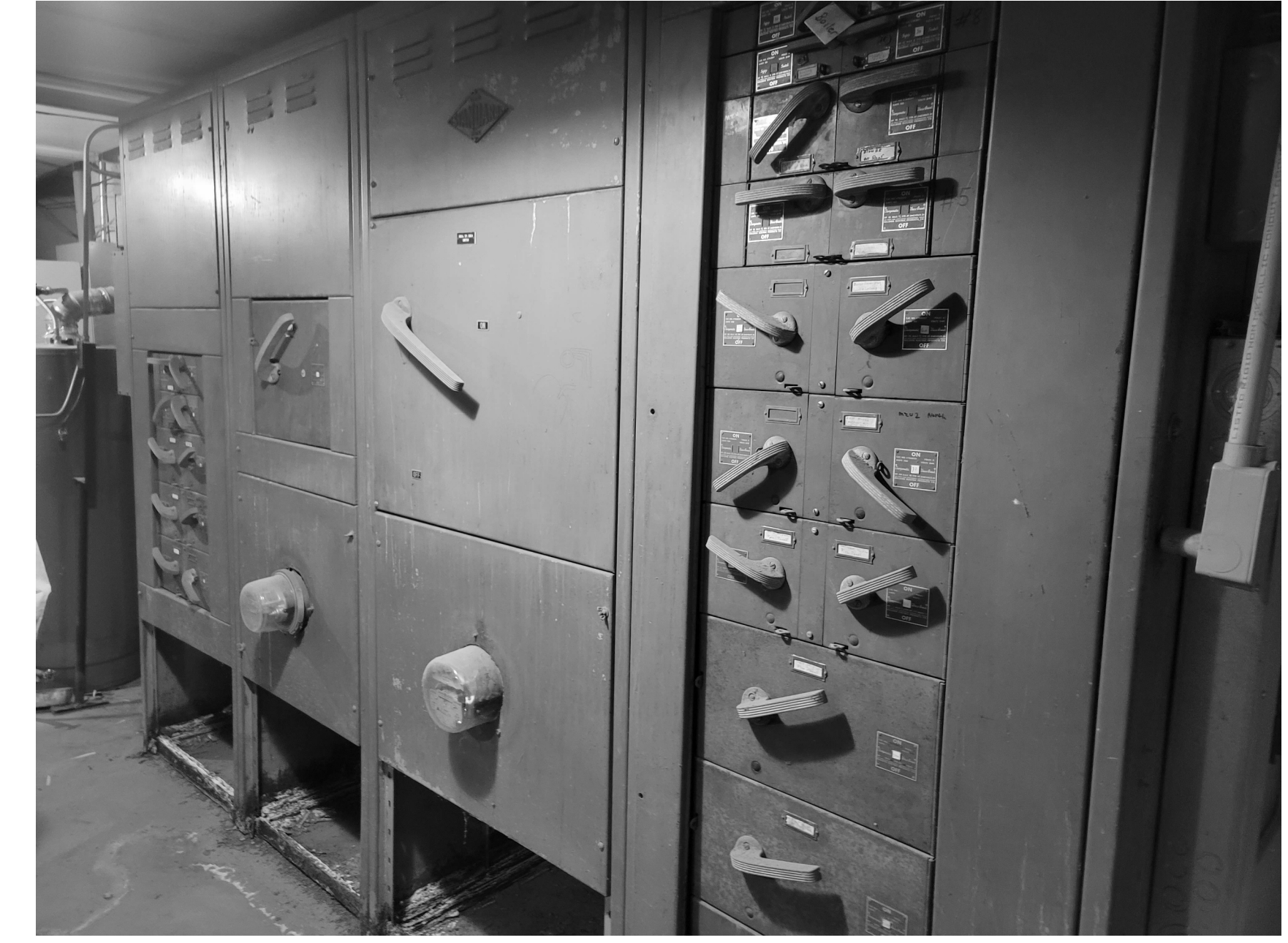
2 EXISTING ELECTRICAL GEAR ES101 NOT TO SCALE
